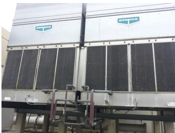
Figure 7: Evapco Cooling Towers
